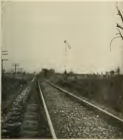
FIG. 5. OBLIQUE POSITION OF SEMAPHORE BLADE, BLOCK IS CLEAR.
